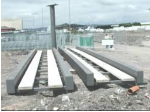
Photograph 5 - Elevated superstructure waiting to be lifted into position
