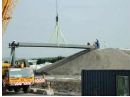
Photograph 6 - Lifting in the elevated sections
