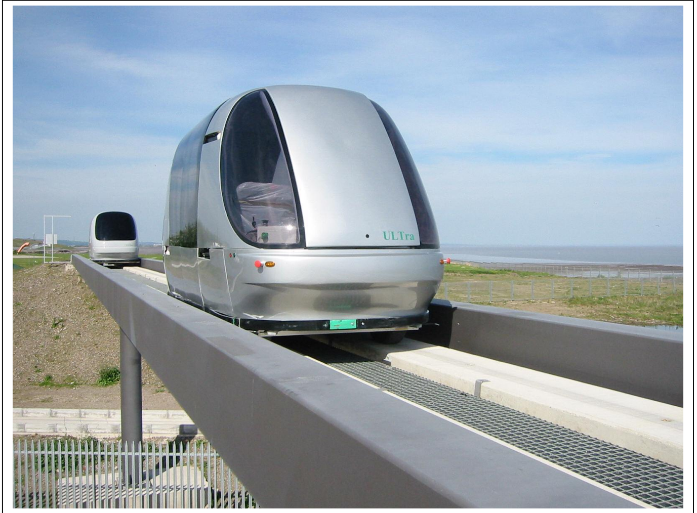
FIGURE 2 ULTra elevated guideway and T-Pods.
