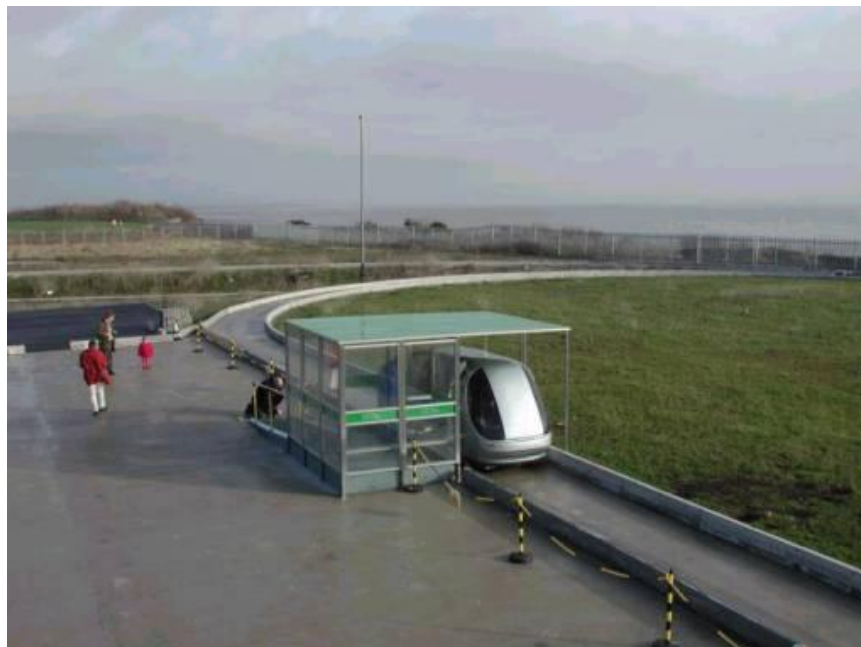
Figure 1 General View of Cardiff Test Track Showing Station
