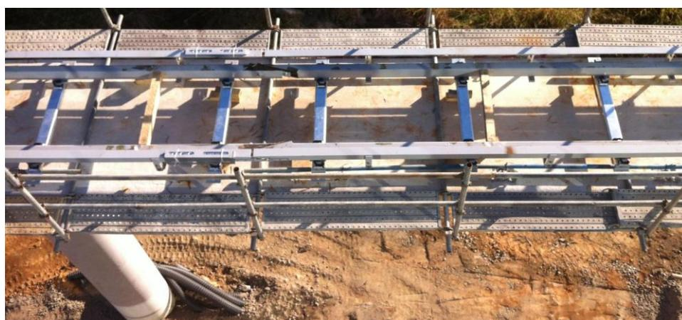
Steel track being laid onto the concrete guideway
