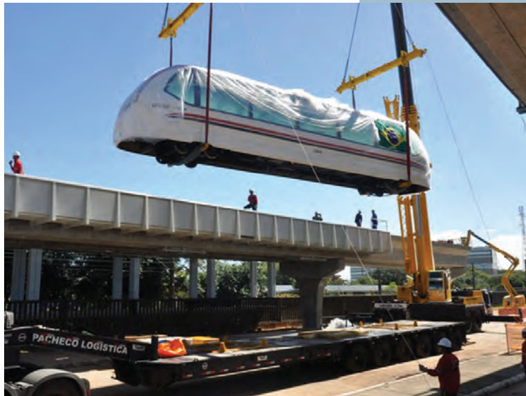
An Aeromovel vehicle in Porto Alegre, Brazil, is lifted into its air-propelling guideway.
