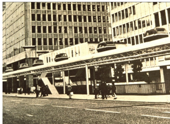
British Cabtrack PRT system.
